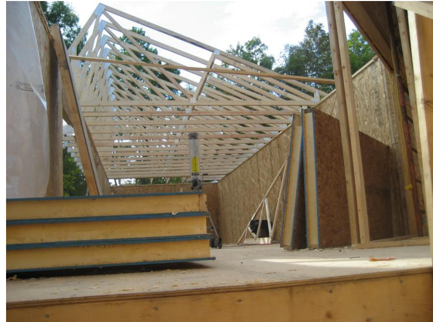
14. Interior View of Roof Installation
