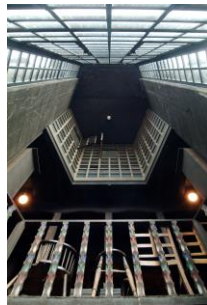
Interior Window Details
