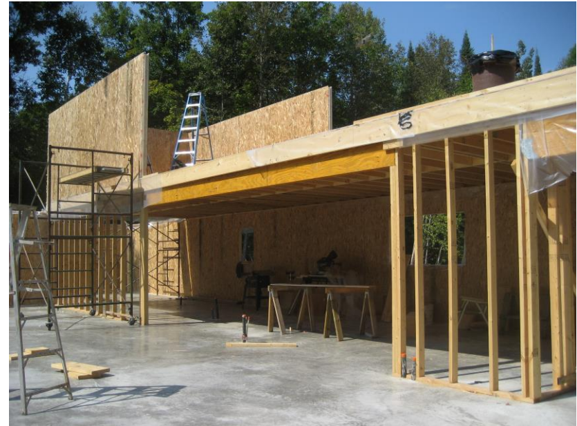
12. Framing second floor
