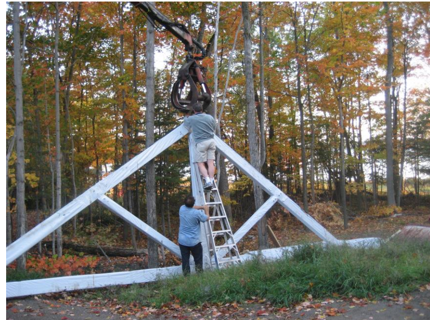
16. Lifting main roof support
