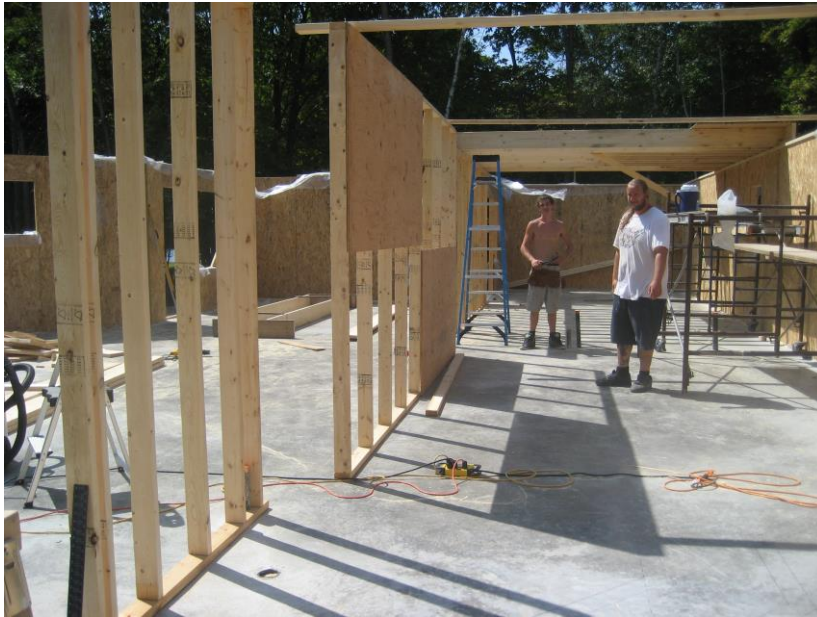
11. Framing first floor
