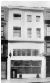
Willow Tea Room Facade
