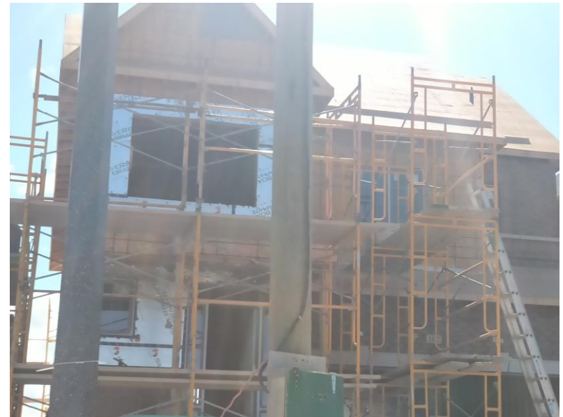
32. Scaffolding for window and door installation
