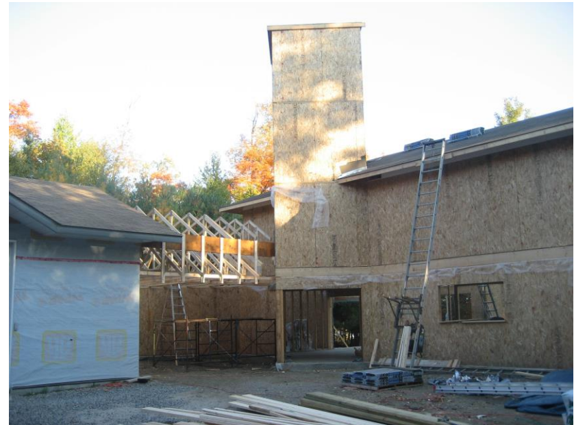
18. Final roof paneling and tower construction
