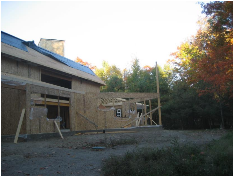
21. Forming architectural feature
