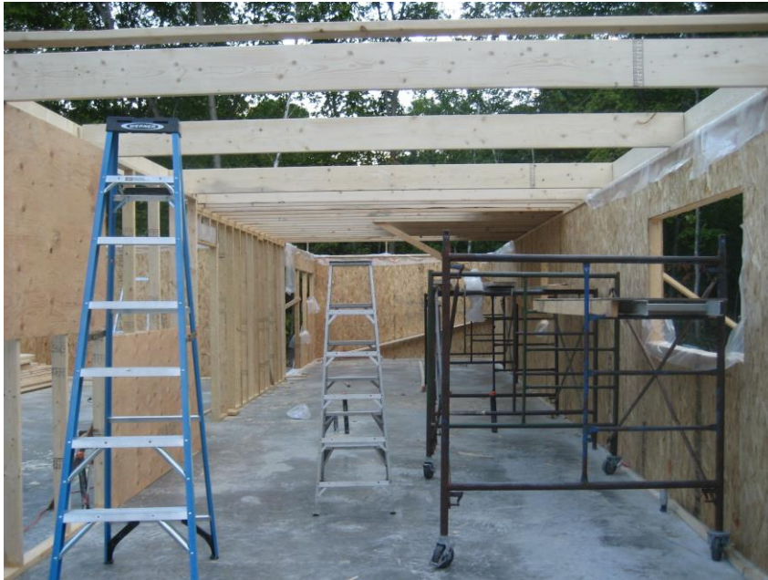
13. Second Floor Joists
