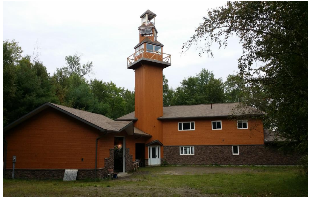
20. Tower window installation
