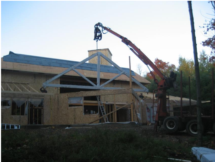
17. Installation for roof support beam
