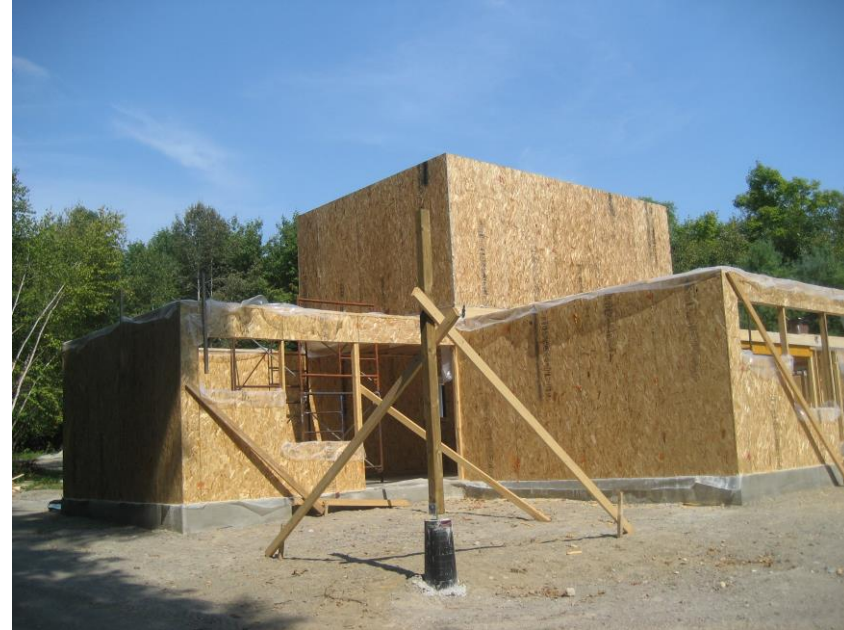
10. Plywood Walls-Exterior View
