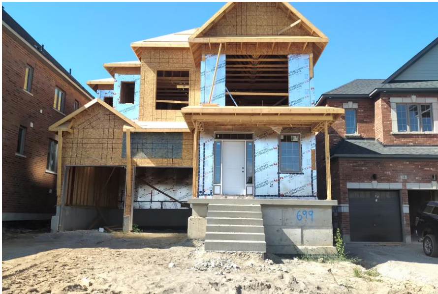
31. Before window and door installation
