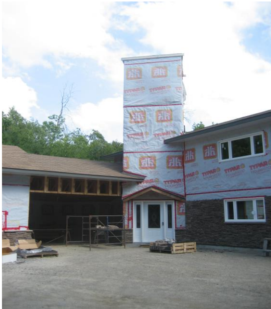
23. Wrapping tower for weather proofing
