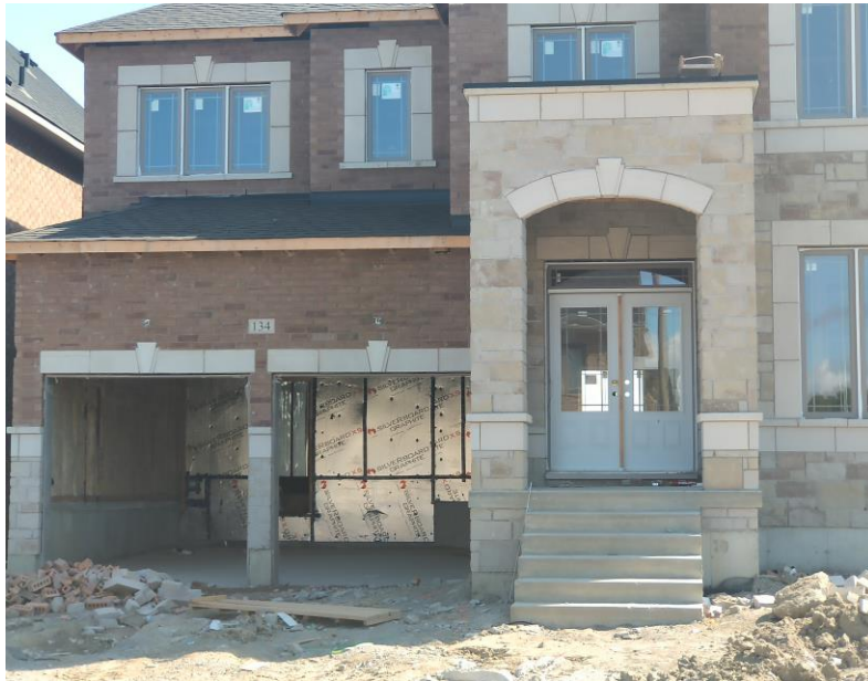
33. After window and door installation
