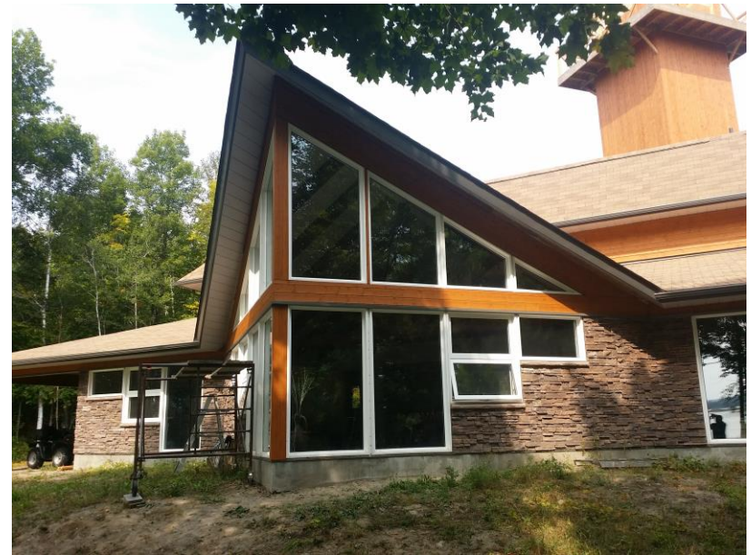
22. Completion of architectural feature
