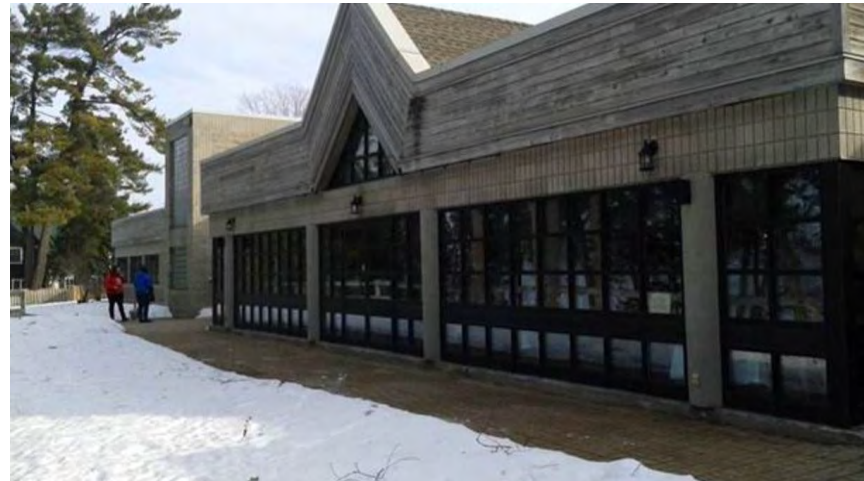
Patio, East View
